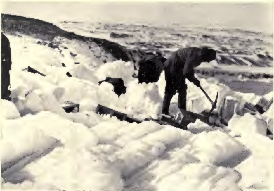
DIGGING OUT STORES AFTER THE CASES HAD BEEN BURIED IN ICE DURING A BLIZZARD
